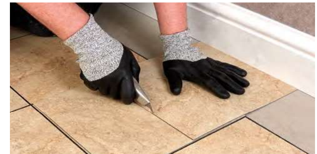
Figure 5.6 Measuring using an overlapping tile
