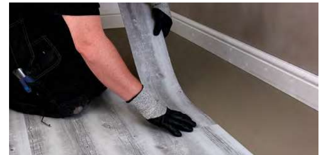
Figure 5.1 Setting planks out
