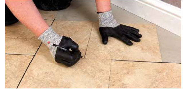
Figure 5.8 Marking using an overlapping template on diagonal laid tiles
