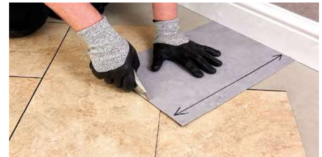
Figure 5.9 Cutting the perimeter tiles (diagonal cut)
